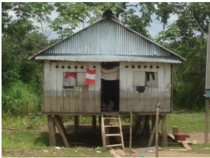
Flood level marks on house in Peru. Discolouring caused by floods in 2012 (upper level) and 2015 (lower level) is visible on this house in Iquitos, Peru. (Photo: Juan Bazo)
