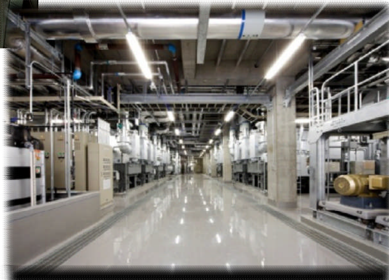
Power Supply and Cooling Unit Building
