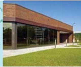
Reston WCOSS Primary Facility
